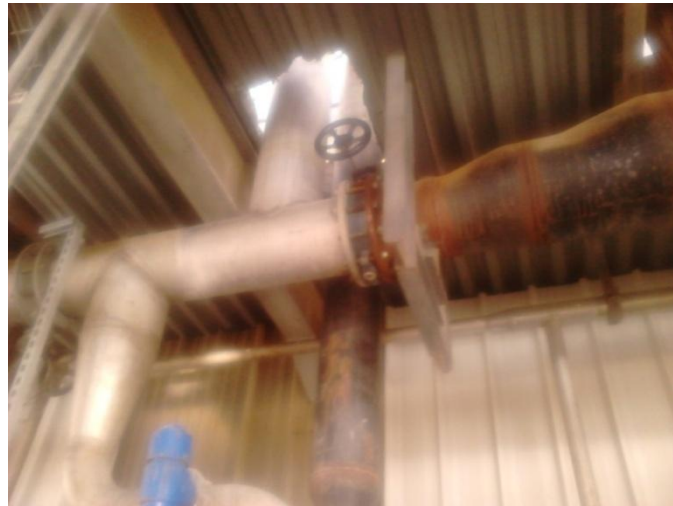
Figure 10 : séparation circuit vide 1
